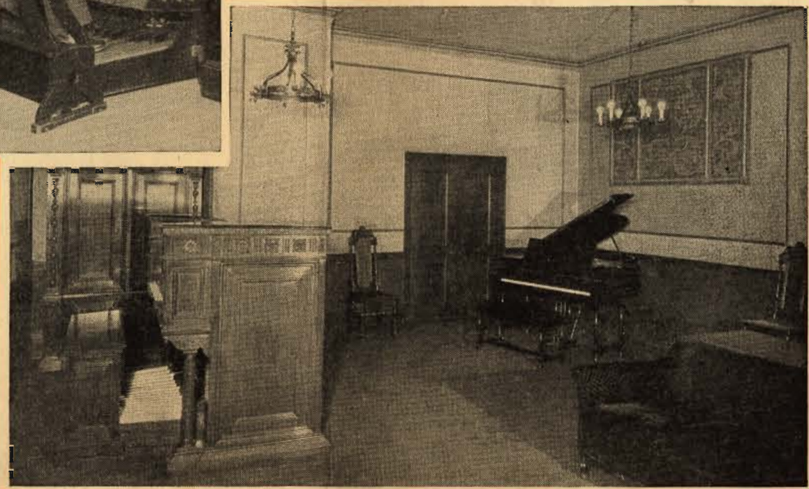
Corner of ORGAN STUDIO. Two Kimball organs are installed.
